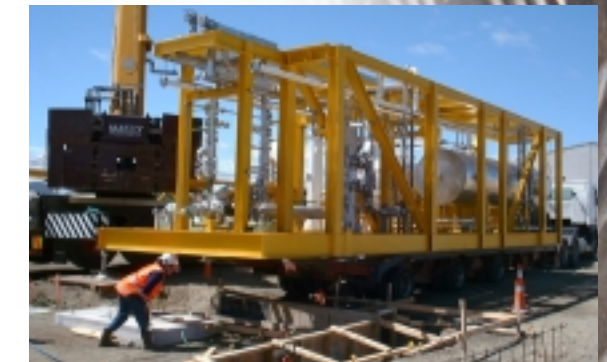
Pohokura Development Mechanical installation, commissioning and joint integrity
