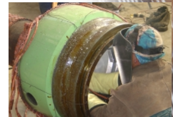
Pipe Casing for Pohokura
